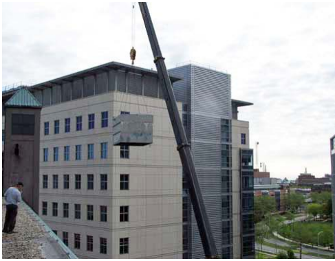
Multiple Tower Replacements
