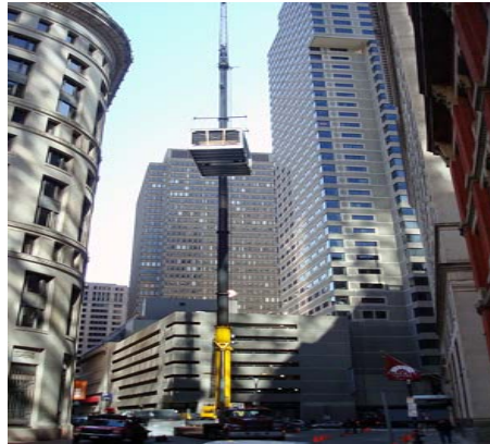
Cooling tower replacement on 18th floor
